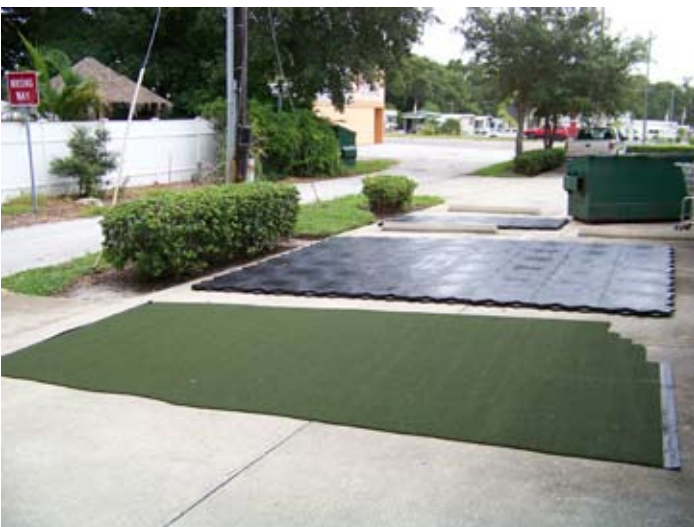
The turf is left next to the panels to ensure same temperatures are achieved prior to affixing the turf to the panels.
