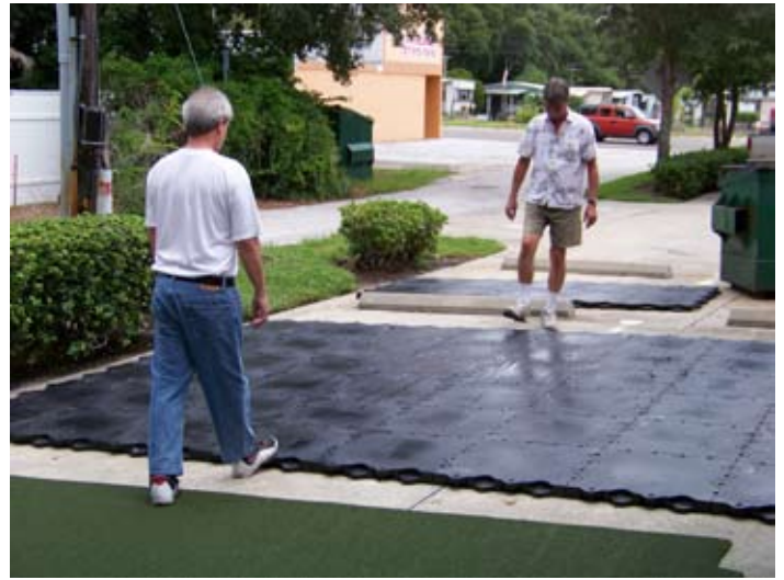
Kick the panels together with one person on either side of layout.
