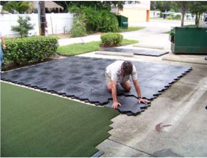
Prepare the ground and assemble the panels as normally done.
