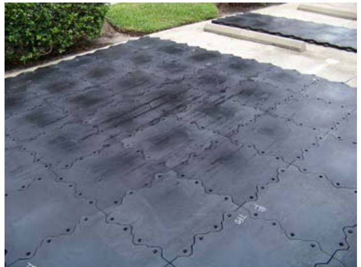
Panels are assembled with no gaps regardless of outdoor temperatures. No screws are used around the perimeter. Stapling the turf to the outermost edges of the panels will hold the entire system in place. If screws are needed over contours to create proper alignment it is O.K. to do so. Belt sand down any high teeth tips on contours.
